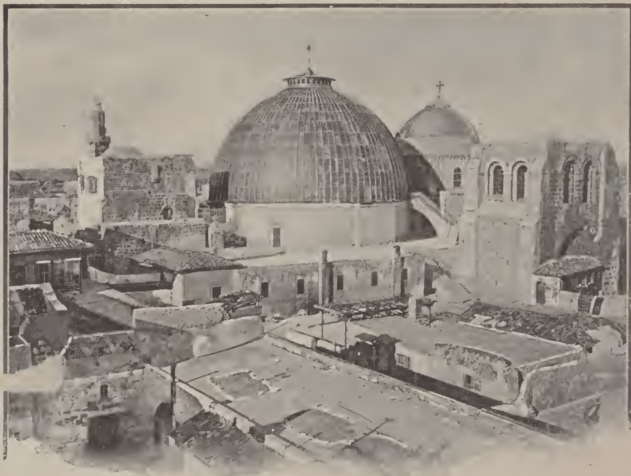
ROOF OF THE CHURCH OF THE HOLY SEPULCHRE.
